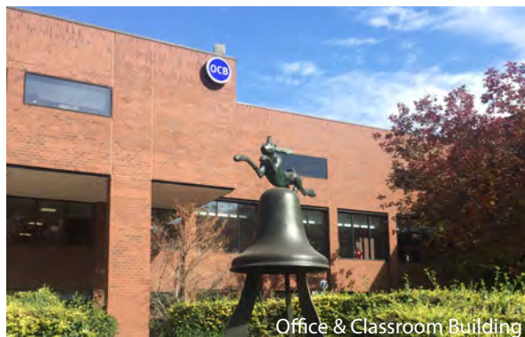
Office & Classroom Building
