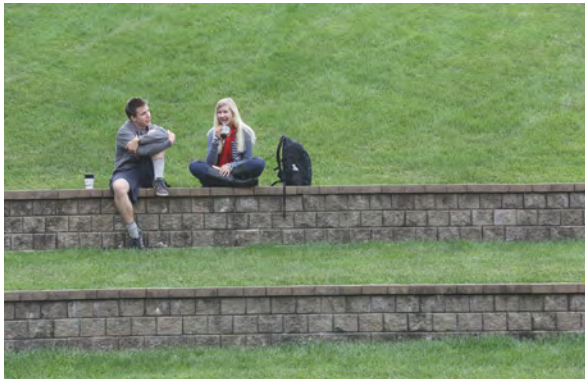
Water Tank Berm
